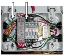
9. Connect green wire to the ground terminal Connect white wire to the N terminal Connect black wire to L1 terminal
