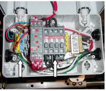
Connect green wire to the ground terminal Connect white wire to the N terminal Connect black wire to T3 terminal (see next page for details) Step 6
