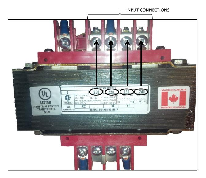
TRANSFORMER OFFERS 4 DIFFERENT INPUT POWER SUPPLY OPTIONS FACTORY SET AT 220V. IT IS IMPORTANT TO CHANGE YOUR INPUT CONNECTION BASED ON YOUR POWER SUPPLY, AS THE BURNER WILL NOT OPERATE PROPERLY
